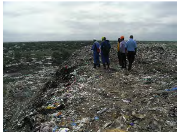
Figure 2. Collapsed cliff of the Hulene dumpsite.
