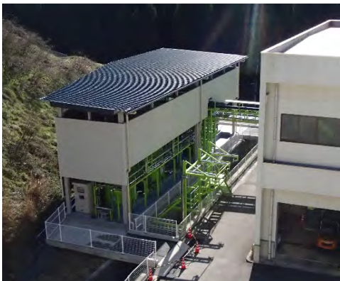
Pic.1 The foreground of eco sodium hypochlorite generating apparatus
