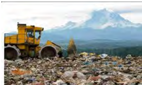
Figure 17 Landfill compactor crushing large waste
