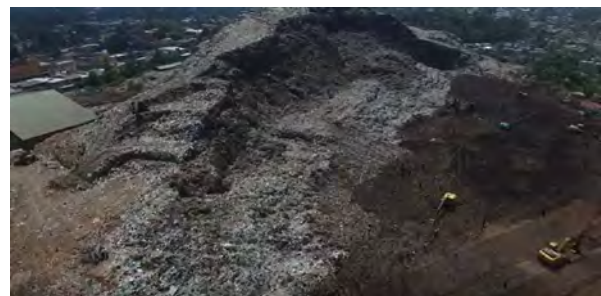
Figure 10. Collapsed cliff and secondary cracks (drone photo by JDR Expert Team, 2017).
