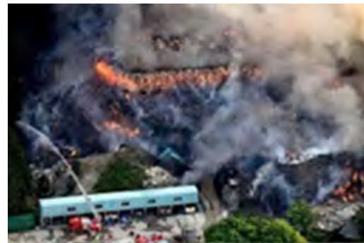
Figure 8 Fire from waste
