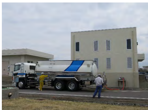
Pic.3 Eco sodium hypochlorite injection equipment in sewage treatment plant
