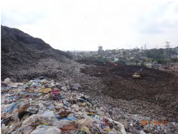
Figure 7. Collapsed cliff and waste debris.
