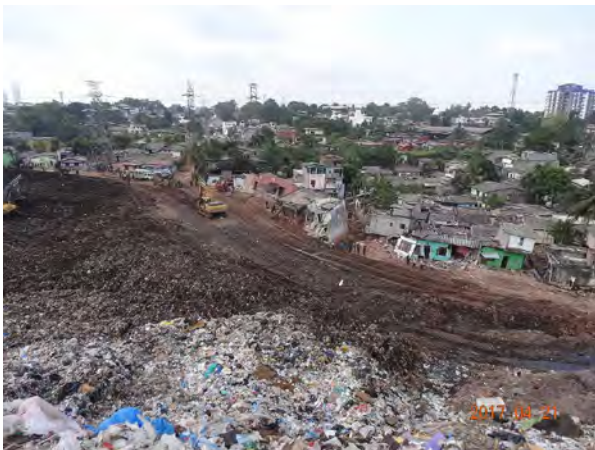
Figure 9. Inclined ground and crushed houses caused by the dumpsite collapse.
